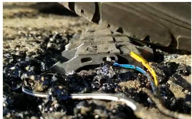
Photos of exposed RPS during operation.
